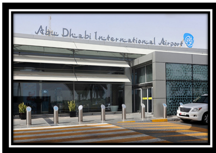
Abu Dhabi Etihad Terminal
